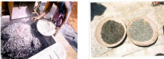
Figure: Mixing of Plastic with Hot Aggregate
